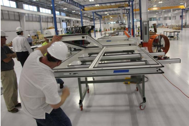
New Hudson Facades is a glass-making business that is an offshoot of real-estate developer Related Cos., which teamed up with a specialty-metal manufacturer so as to ensure a supply of glass panels. PHOTO: ROBBIE WHELAN/THE WALL STREET JOURNAL
